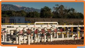
Dupont terminal was recently upgraded in 2Q 2017. This included an upgraded three-bay loading rack and additive system as well as TAS installation. An Ethanol automation project is in progress with a completion date of mid 2018.
